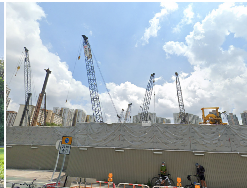
LR1.3 CONSTRUCTION SITE
